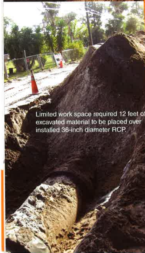
36-inch diameter RCP installed to Standards with compaction to spring line and finished grade
